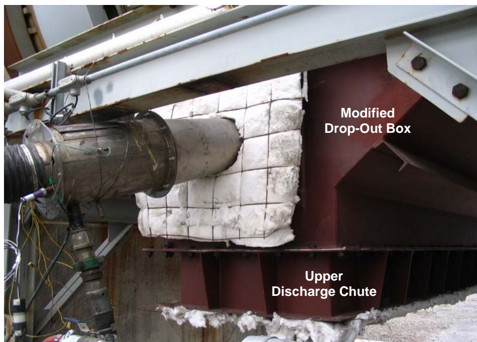
Figure 3. TEAM's 10-Million Btu/hour Burner Installed and Insulated in North Drop-Out Box Access Hatchway
