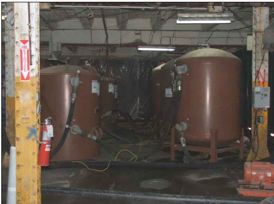
Photograph 12 Wastewater Treatment – Carbon Filters
