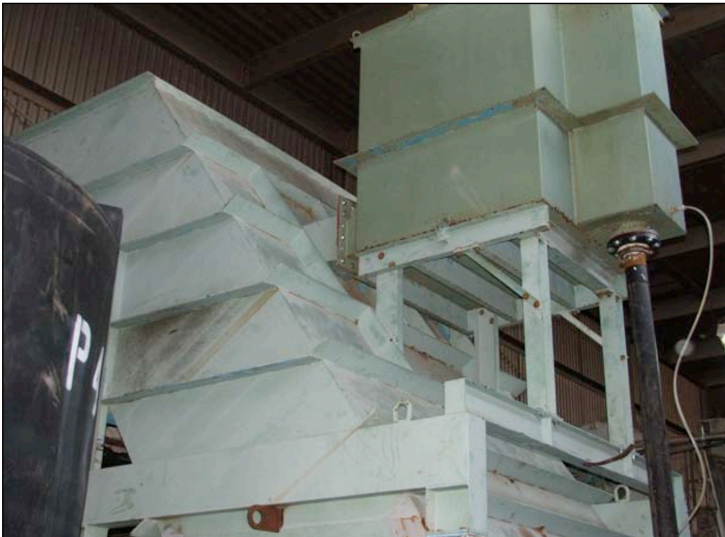
Photograph 10 Wastewater Treatment – Clarifier
