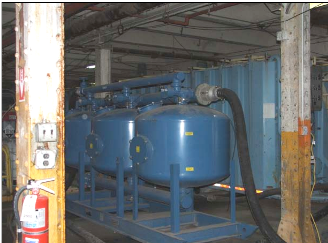
Photograph 11 Wastewater Treatment – Pressure Filters
